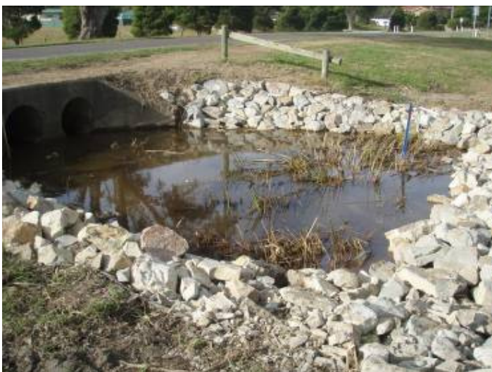
One of the five sediment dams which have been constructed along Bullara St. Pambula
